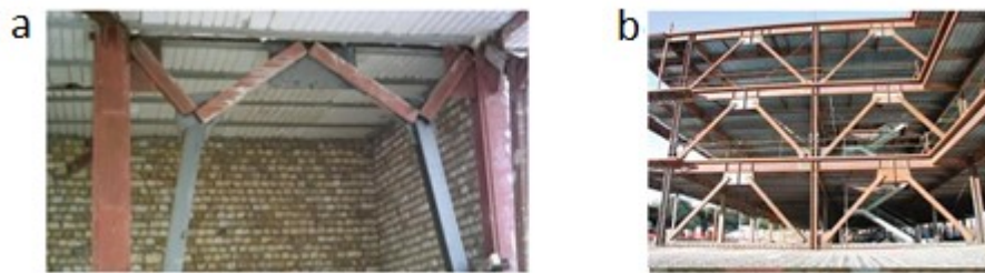
Fig. 1. (a) Gate brace [15]; (b) Inverted V brace [17].
