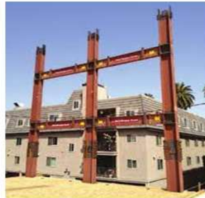
Fig. 4. (a) FE model in the present paper with ABAQUS software; (b) SMF manufactured by PACO Engineering Company [28].
