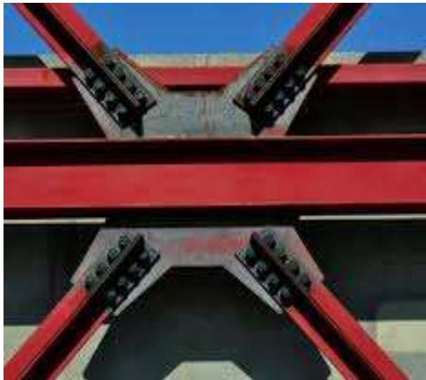
Fig. A. Smart Steel Braced Frame by PACO Engineering Company in USA [29] (a) column-ground connection; (b) brace-frame connection [29]; (c) beam-column connection[29]; (d) brace-beam connection [29].
